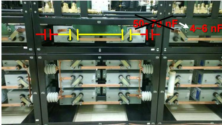
Figure 16. Isolating PEBB capacitors
